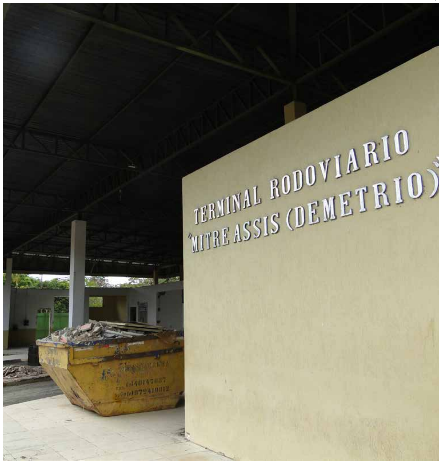
Terminal Rodoviário Municipal "Mitre Assis"
